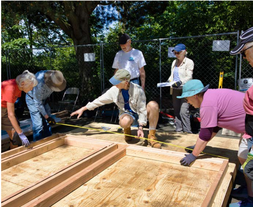
▲ The Saint Mark's Habitat for Humanity crew constructing a tiny house in the cathedral parking lot, June 8, 2024.
